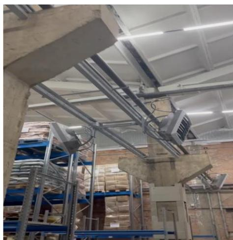
Picture 3 - Location of air-heating units
