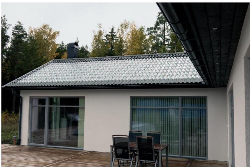
Figure 1. View of a house with glass roof tiles.
