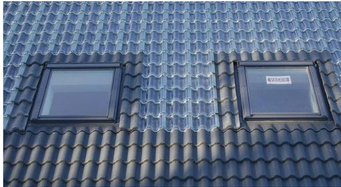
Figure 2. Combination of glass and conventional roof tiles.
