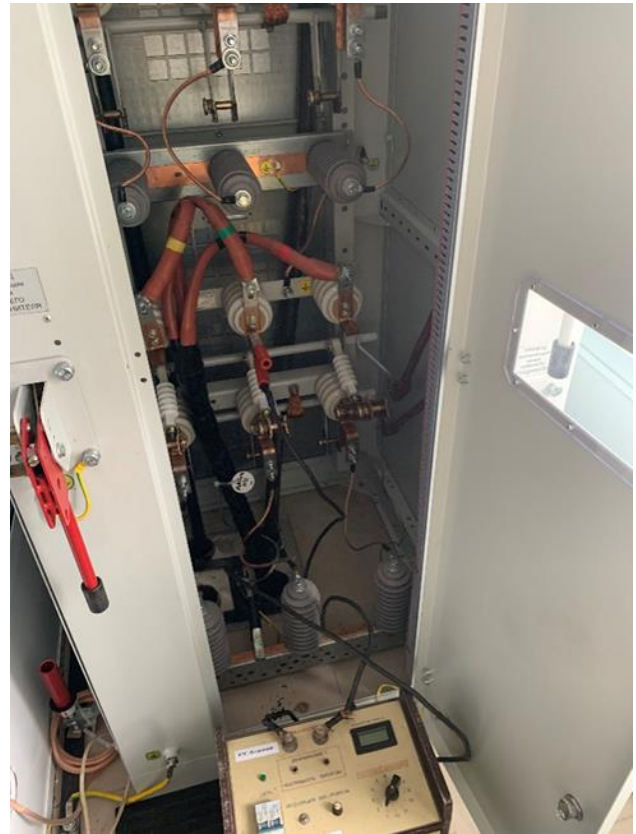
Fig. 7. Connection of audio frequency generator to AABl-10 3x95 cable
